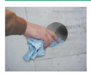
Before installation the **MASTER-RING** gasket insert, the inside of the core drill hole and the outside of the gas, water, sewage pipes as well as the cables have to be cleaned.
