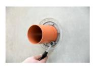
Tighten the screws crosswise through one turn.
