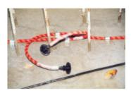
Successive injection hose sections <u>must overlap by at least 20 cm</u> in order to ensure continuous injection of the joint.
