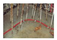
All changes in direction must be implemented with a sufficiently wide bending radius in order not to damage the hose/restrict the overall injection flow.
