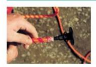
After the hose has been cut to length, screw the respective connecting pieces fully into the hose (as far as they will go) - the image shows our fastening packers.
