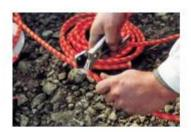
Bind the hose with filament tape and use a suitably sharp tool to cut the hose to the required length. Injection circuits must not exceed 8 m in length.
