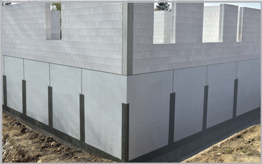
Sealed horizontal and vertical joints
