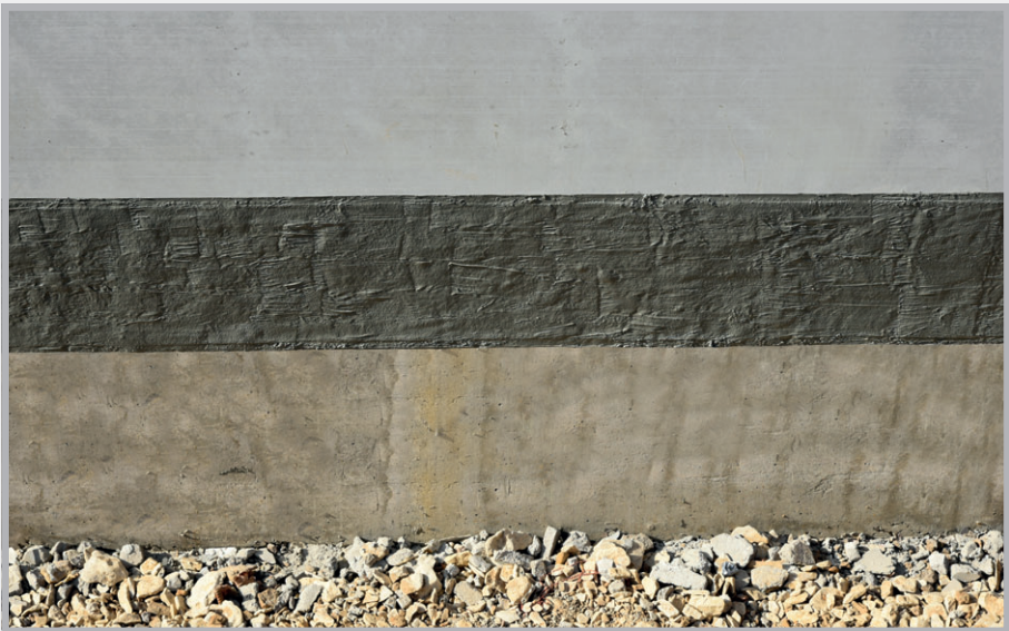
Sealed horizontal joint
